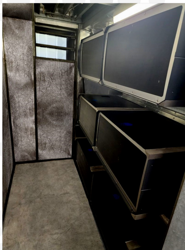
Figure 2. A Bank of 5 MMD-600 Plasma Shield units substituted for the MERV-13 Filter.
